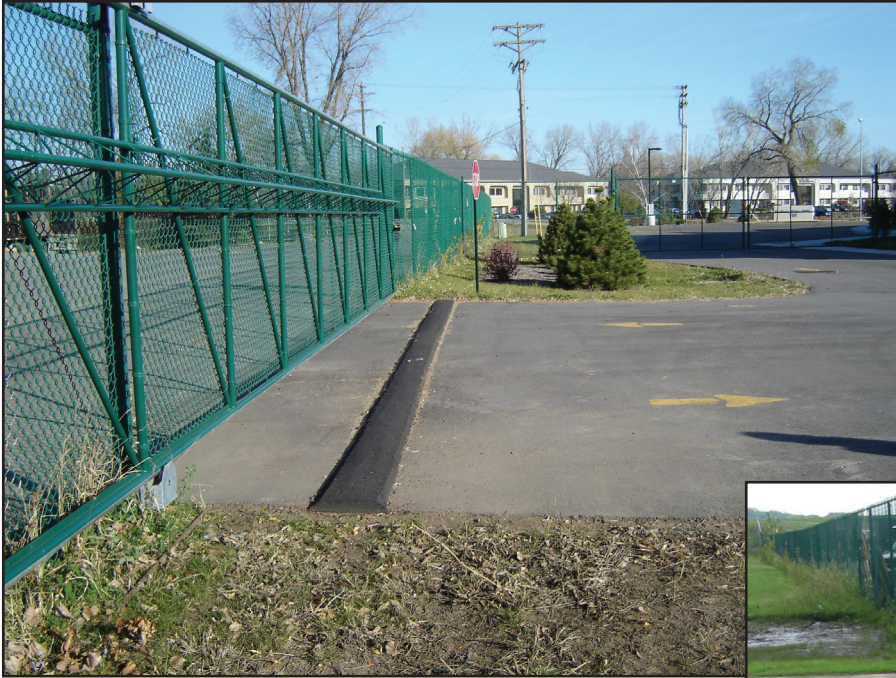
Figure 6. Watershed barrier (speed bump) installed to prevent runoff from City of Madison recycling facility (fenced area to left of photograph).
